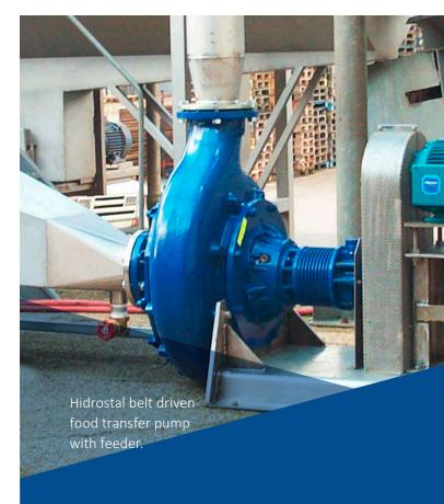
By installing a Hidrostal F-line food transfer pump a reliable continuous process can be established with gentle handling of your product. A closed cycle improves Health & Safety additionally.
