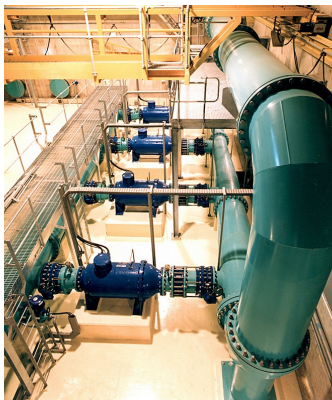
Space saving, noise reducing, flood-proof inline pumps
